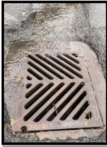
Figure 1-1. Stormwater runoff flowing into a storm drain before making its way to the Skagit River
